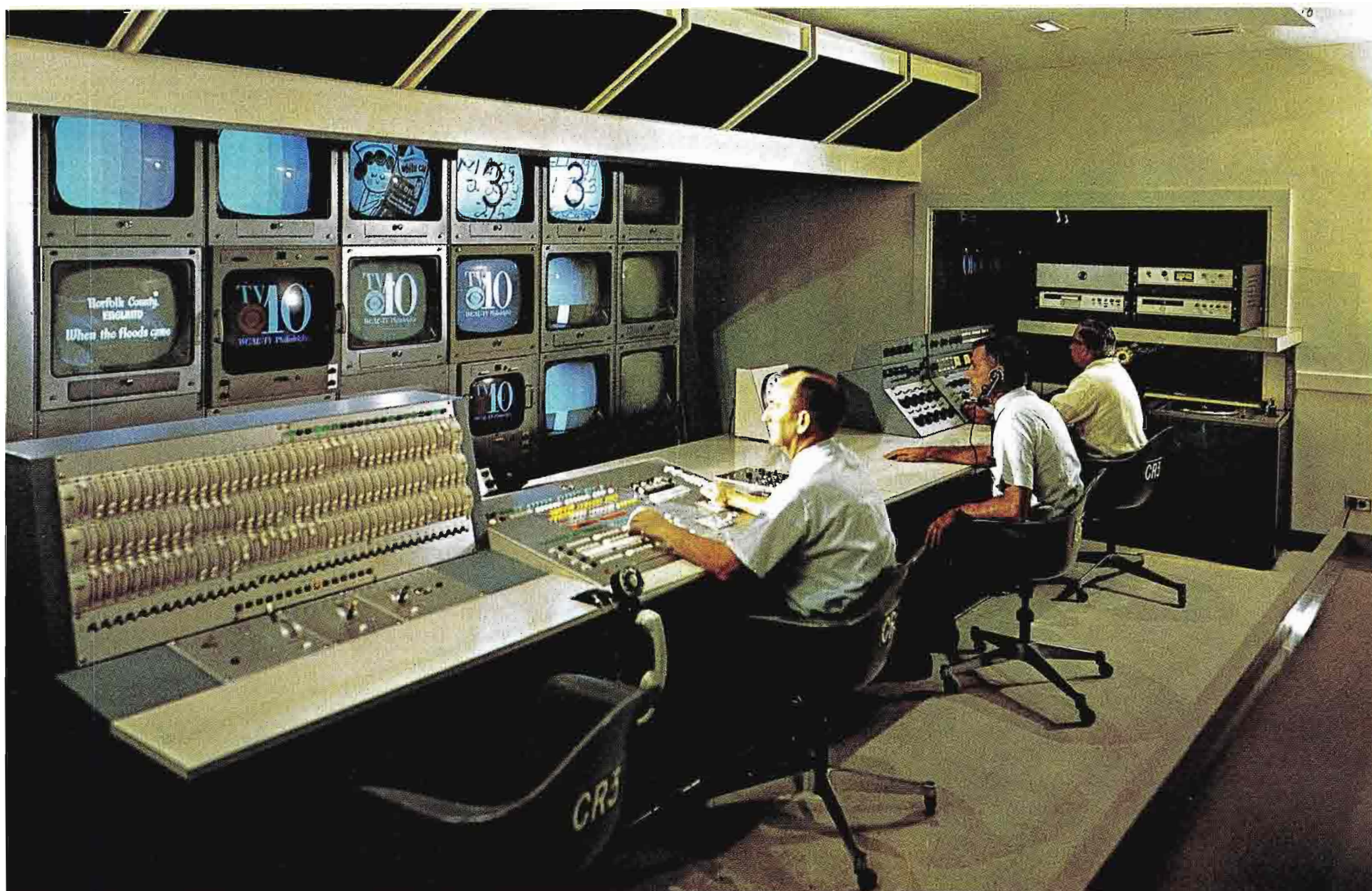
FIG. 6 Studio control room—console contains 3-scene preset lighting control, video switching, director position and audio control (identical for two studios).
