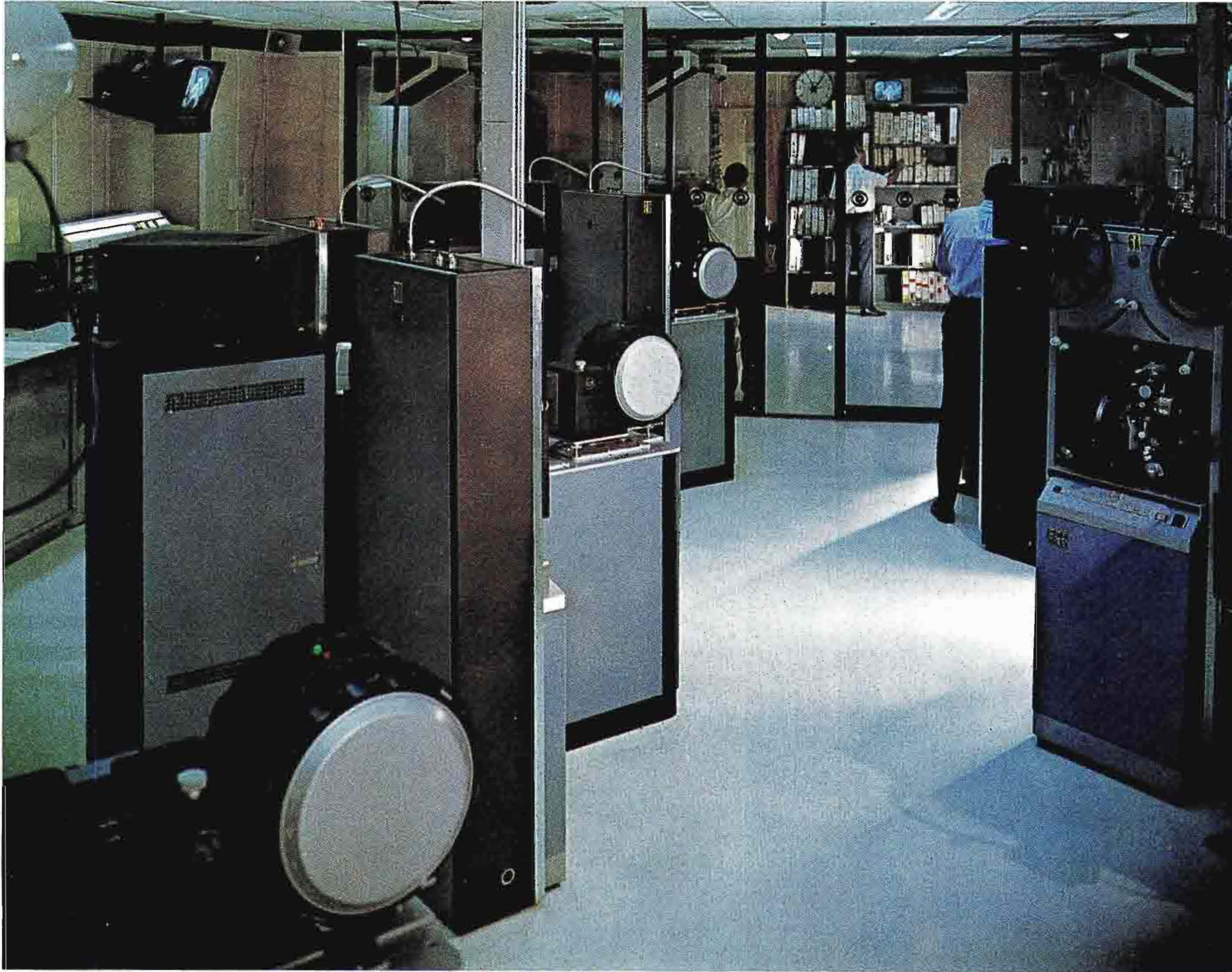
FIG. 3 Telecine consists of six color film islands. Each is multiplexed with two 16mm projectors and one 35mm slide projector.
