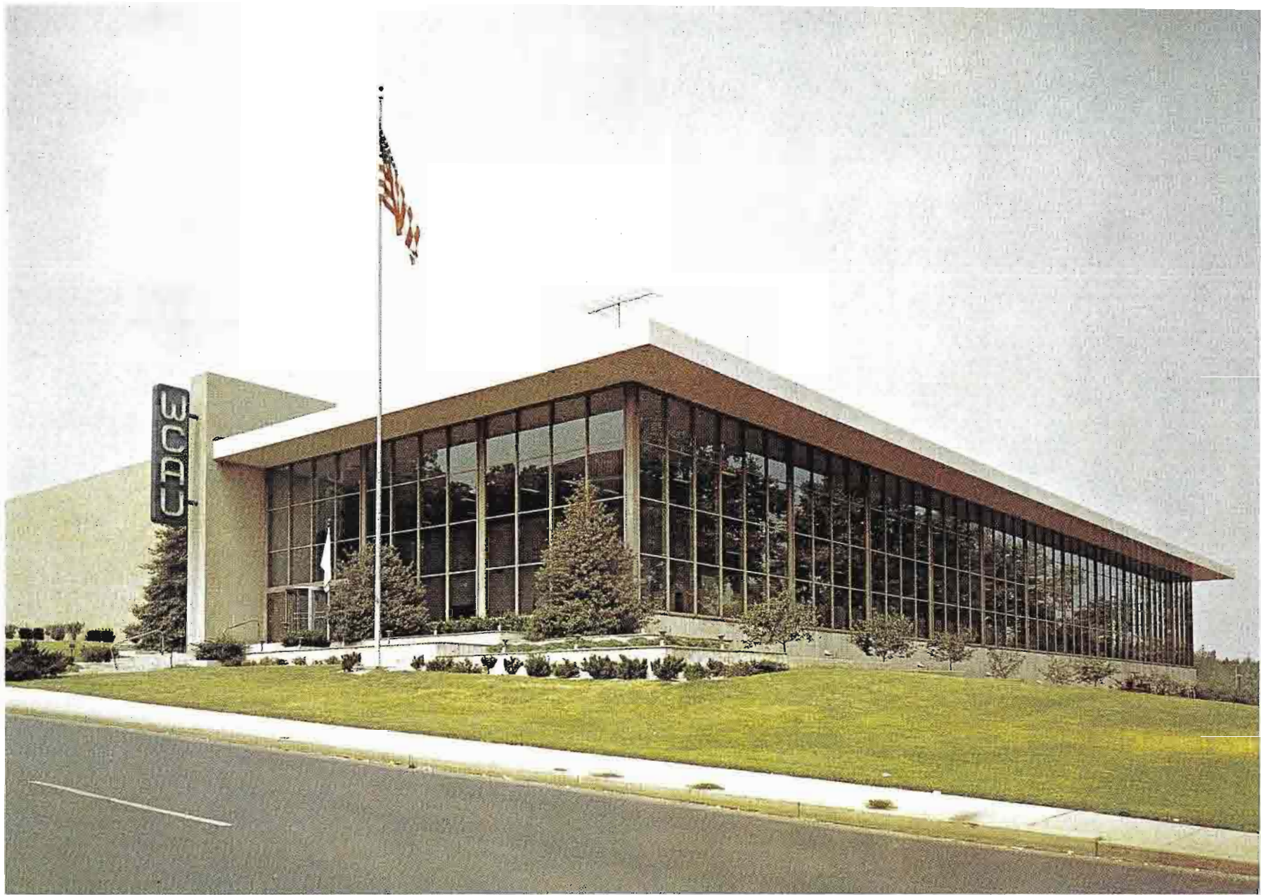
FIG. 1 At City and Monument Avenues in the Philadelphia area, the WCAU-TV building houses a most modern television broadcast center.
